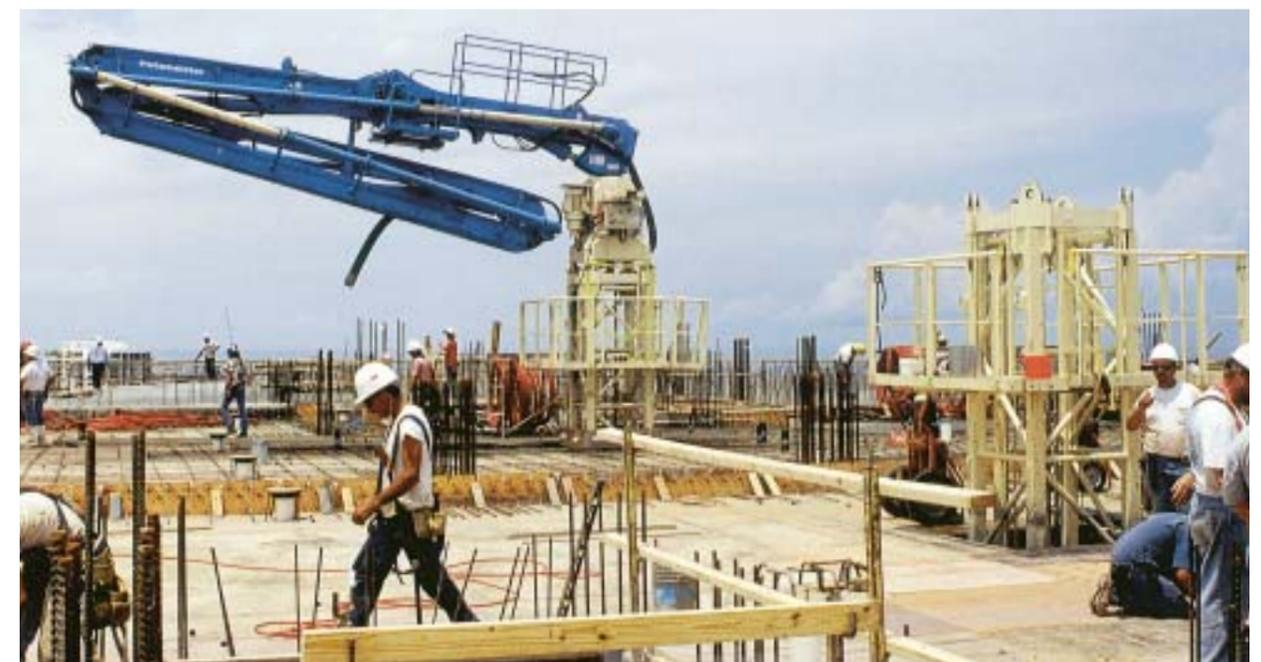
PM satellite system – a placing boom switches between several base structures
