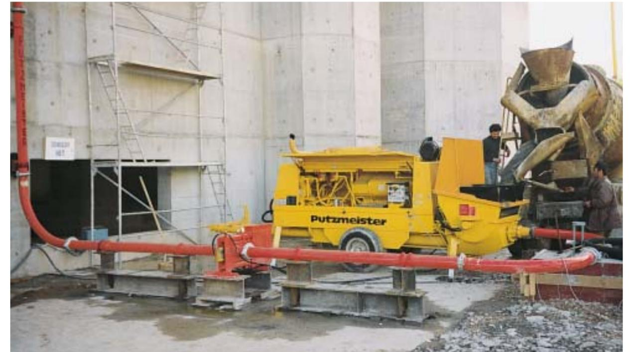
The complete system for concreting and cleaning: know how, concrete pump, pipeline and boom
