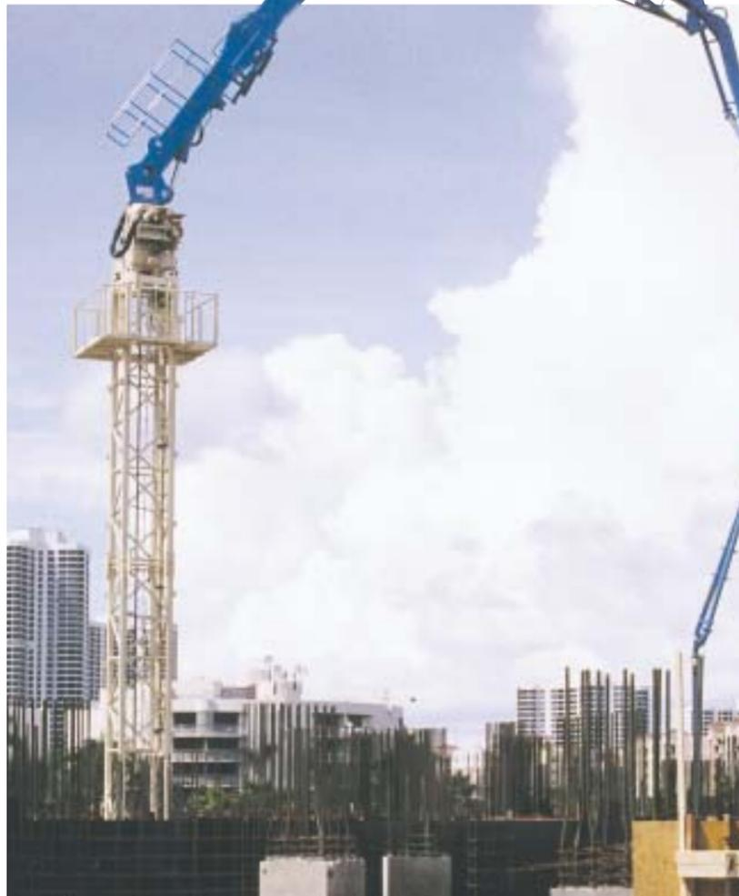
The working platform at the top of the lattice tower facilitates maintenance work as well as assembling and dismantling the placing booms
