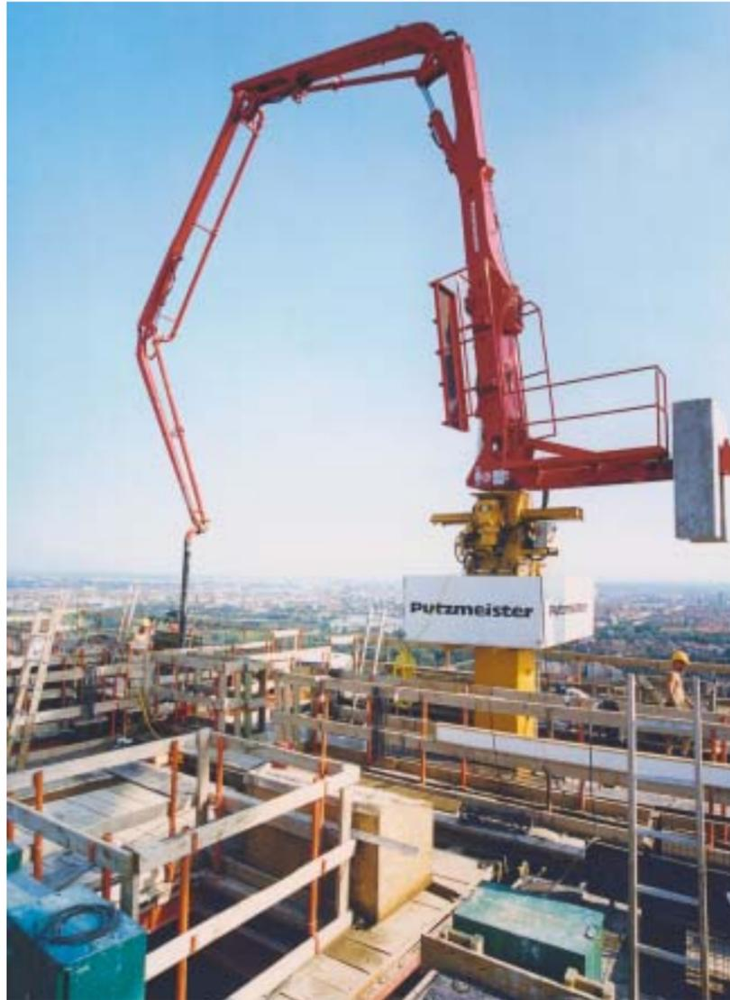
The working platform (A) fits together and surrounds the head piece of the tubular column base structure. It acts as a platform when connecting the boom, allows access during installation and ensures that the areas being concreted can be viewed.
