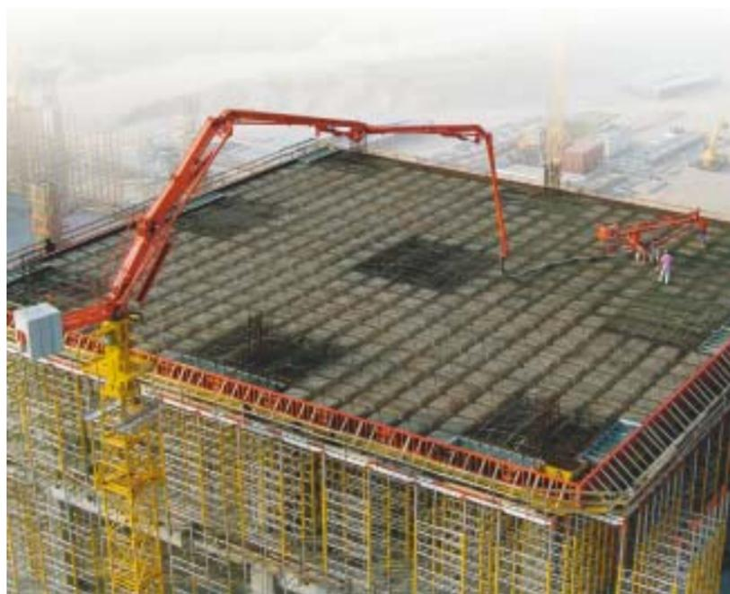
MX 32 on a lattice tower with rotary distributor to increase range
